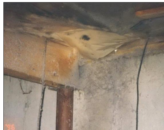
Lint from dryer vented into crawl space; moldy insulation was present.
