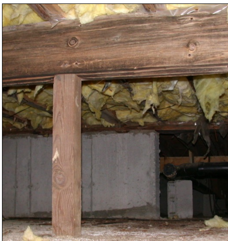
Beam decay due to moisture from dryer vented into crawl space. The top of the post penetrated the bottom of the decayed beam.
