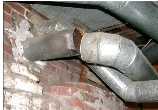
Fallen oil-furnace vent pipe in another house with unhealthy air May Indoor Air Investigations LLC
