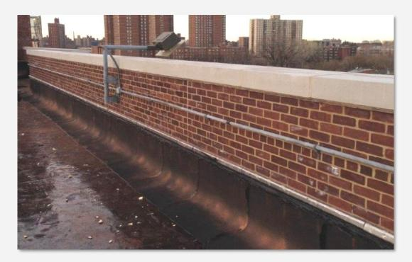
One building science author explains that historically parapets were installed for fire protection. There is a technical purpose of a parapet, to protect the roof edge from uplift wind forces. When wind blows against a building it produces vortices at the roof edges that create huge pressure differences at roof perimeters that can suck roofs off buildings. Parapets dramatically reduce these pressure differences at roof edges.
